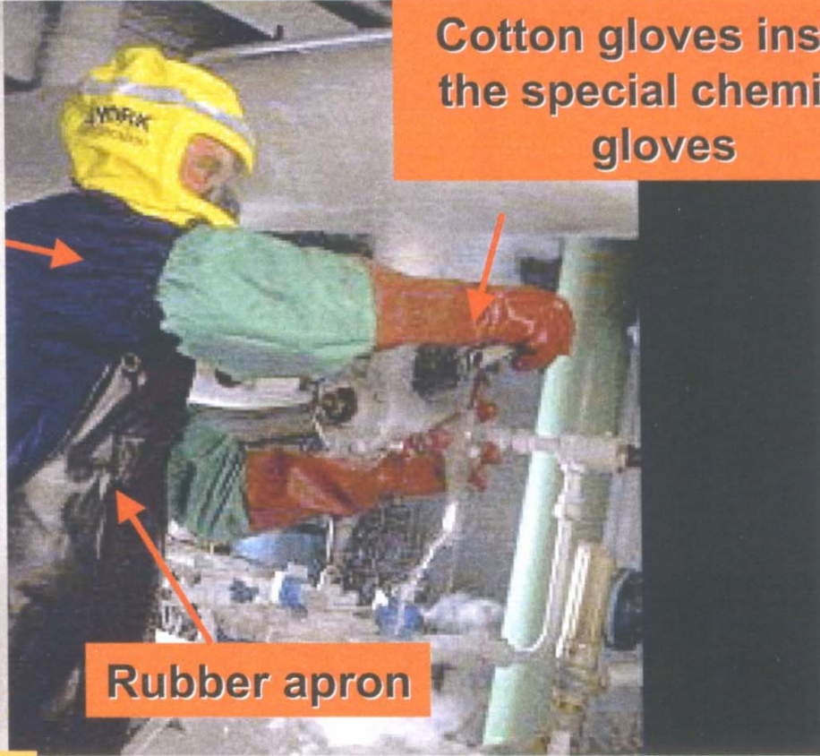
Example of draining an ammonia sample
