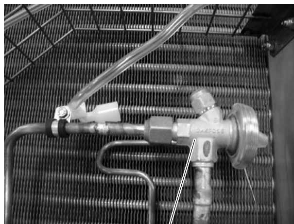
Figure 2-9 Thermostatic expansion valve
